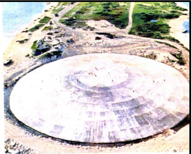
Potential hazard: The concrete dome used to cap off waste from nuclear tests on Runit Island. — AFP
